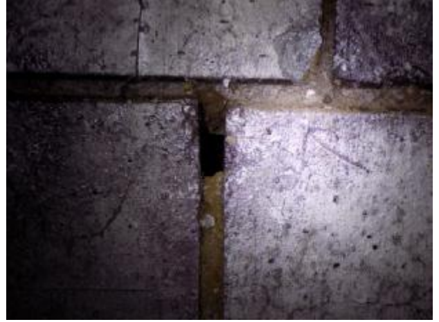
Missing mortar
