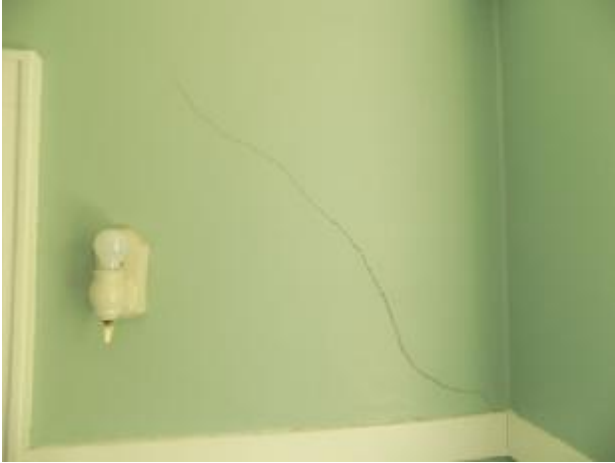
Settling crack
