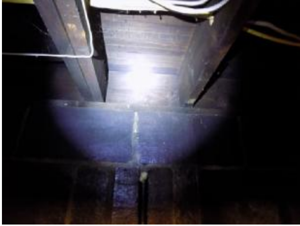
Missing insulation
