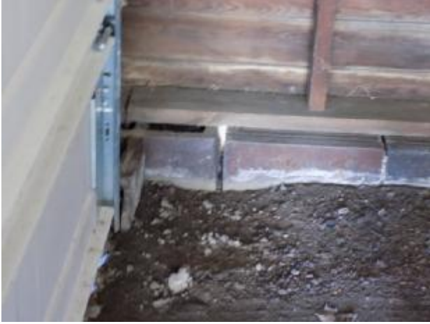
Foundation separation
