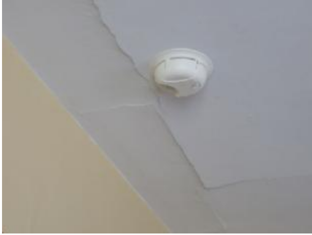
Settling crack
